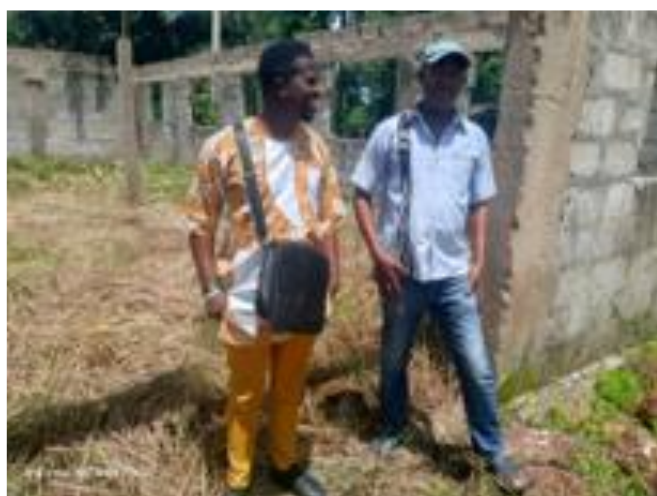
Contractors discussing plans for the Community Centre
