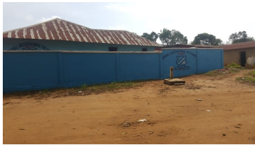
The new wall
