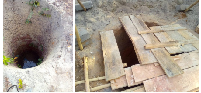
Well at Goshen under construction
