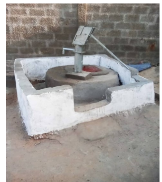
The finished well with new pump
