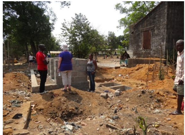
Inspecting the building of toilets 2015
